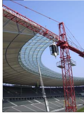
Olympic Stadium Berlin Roof construction
