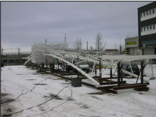
Welding monitoring on a pedestrian bridge (S 690)
