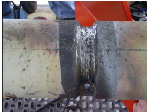
Welding monitoring on a pedestrian bridge (S 690)
