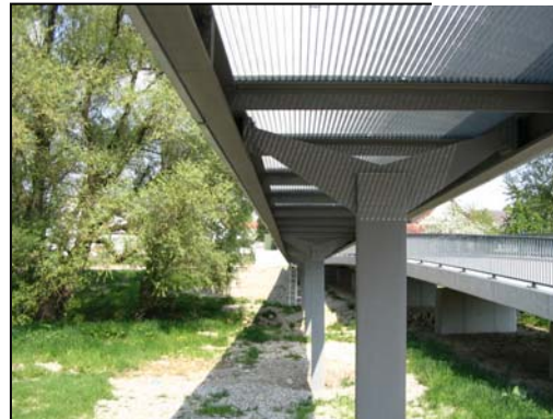
Pedestrian bridge near Ingolstadt
