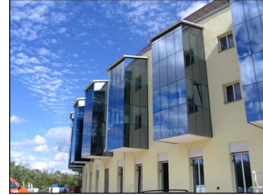
Structural glazing facades
